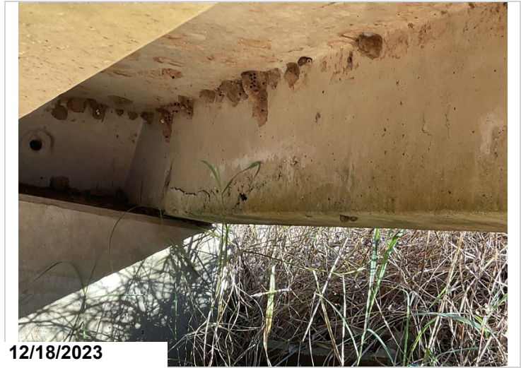
Span 3 unit 6 has delam in right leg near bent 4.
