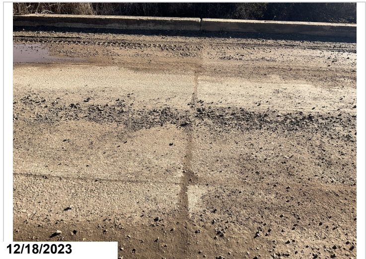
Bent 3 joint seal has debris impaction.
