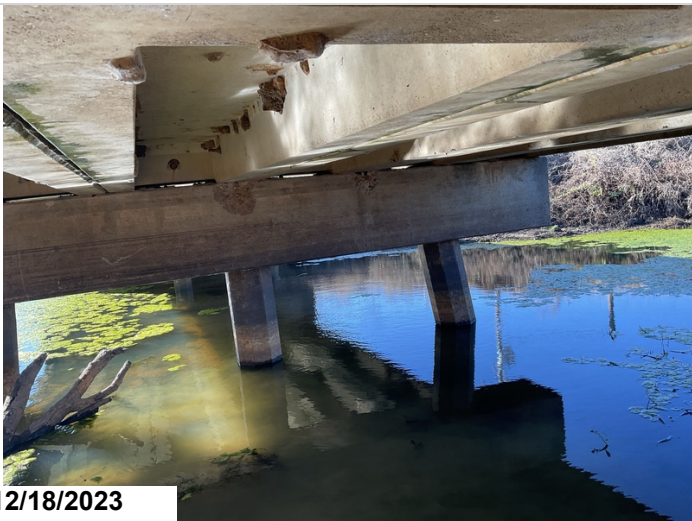
Bent 3 cap ahead has contact spalls.
